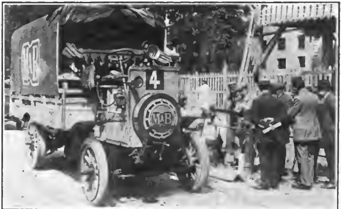
Mallet-et-Blin truck being weighed on the scale at Meulan
